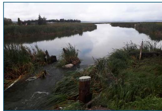
Photo 3: Remains of the old weir, August 2018.
