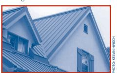
Metal, tile, asphalt, ULC-rated treated shakes or non-combustible material (0 pts) - the most fire resistant and remain effective under severe fire exposure.
